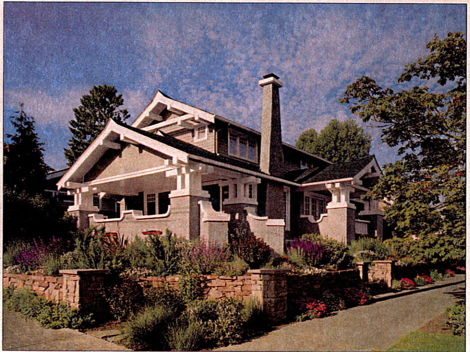
The new second story, containing master bedroom, reading room and bath, fits seamlessly on top of the old house, with a roofline echoing the distinctive pagoda style of the main floor.
